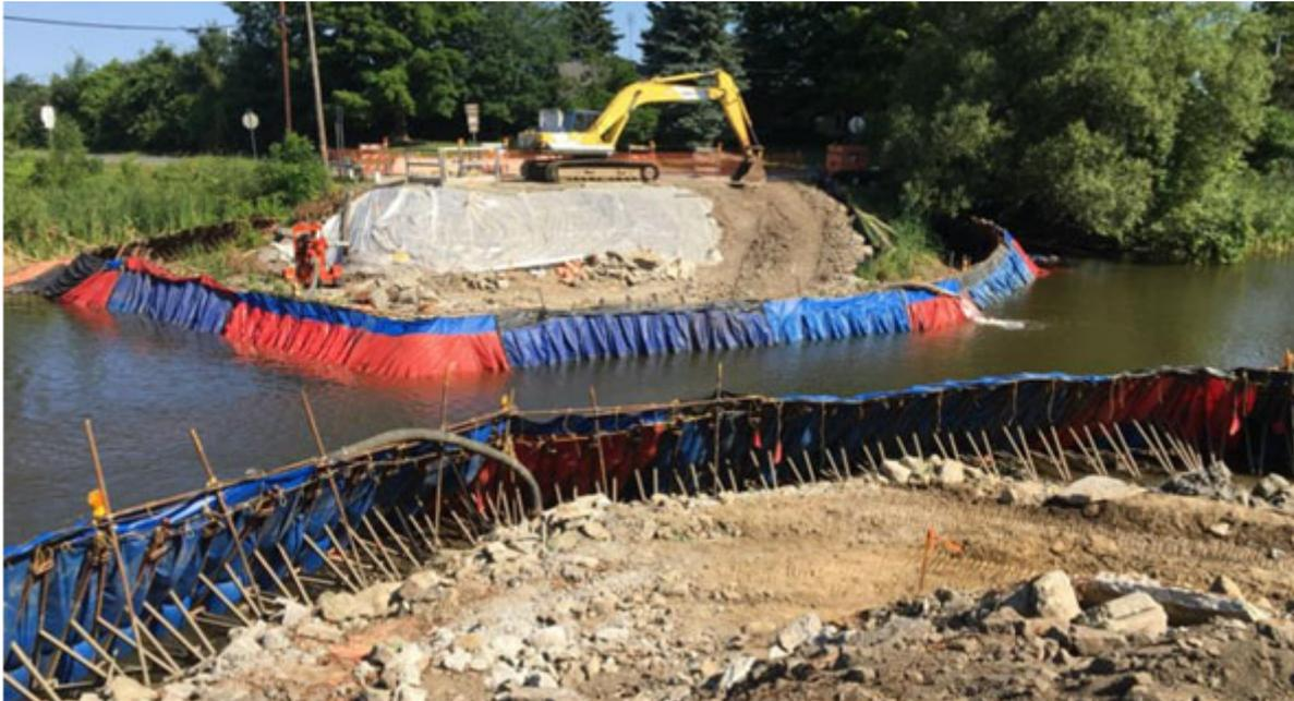
**Figure 2.4: Example Cofferdam<sup>3</sup>**
